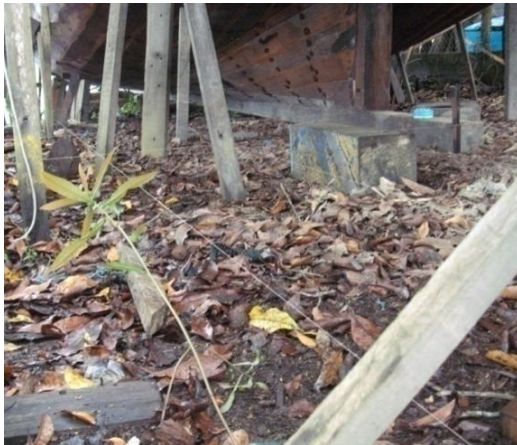
Photo 3.3. Closeup of string grid
