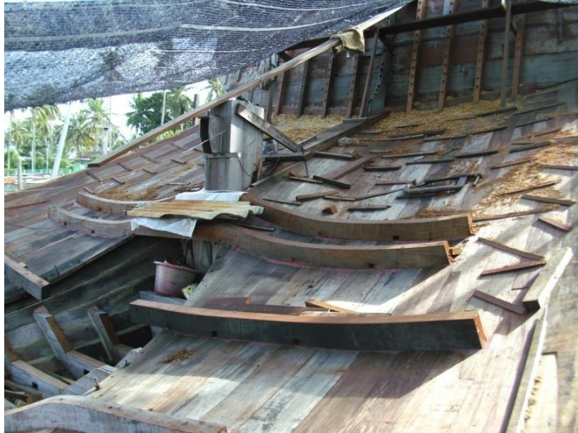
Photo 4.64. 30 m trawler construction showing omega ( \omega ) stern details. Tumpat.
