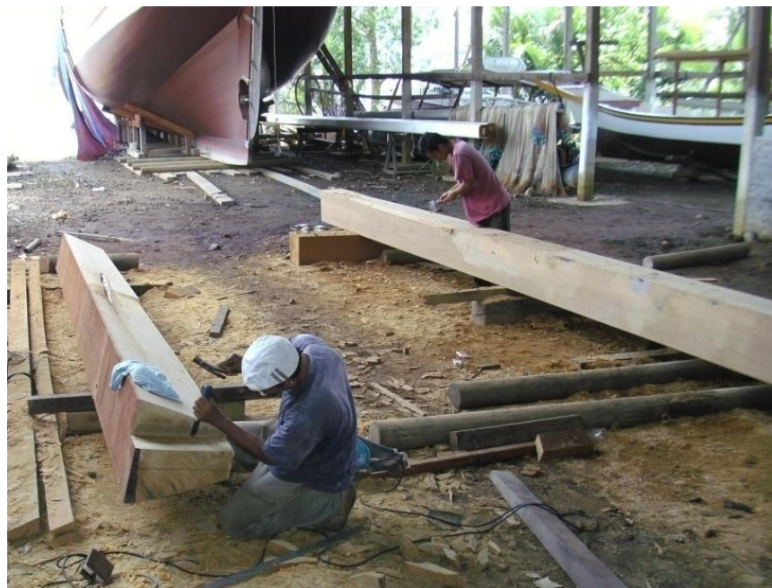
Photo 5.4. Shaping stem post and keel bar. Kuala Terengganu.
