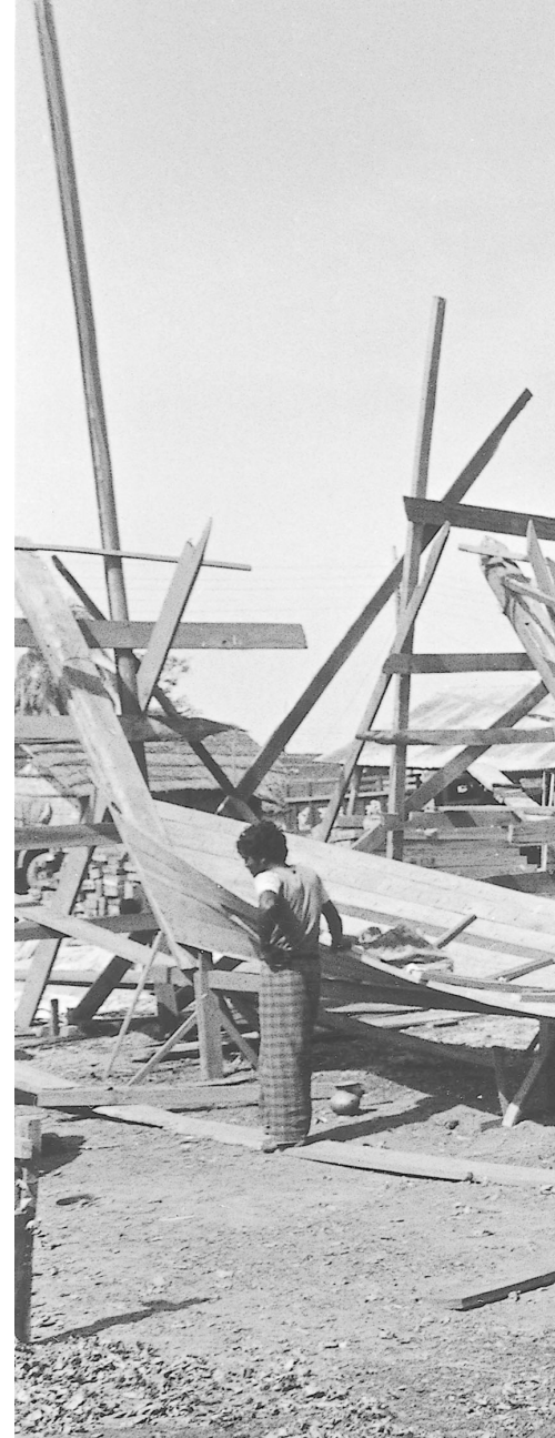
Chandi under construction at a yard in Bangladesh. ▶
