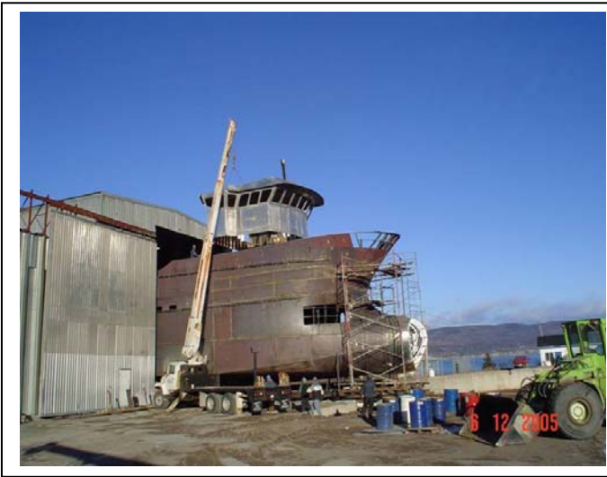
Figure 14: 30.5m (100ft) vessel with bulbous bow under construction
