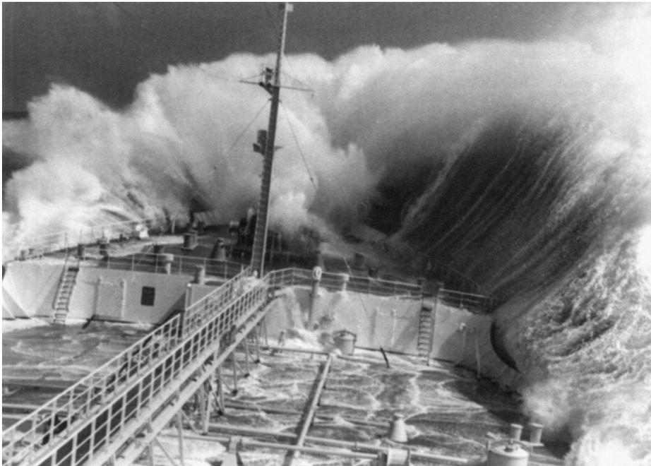
Figure 8.36. Illustration of green water when the tanker *Siri* met Typhoon Judy southeast of Okinawa in 1963. The relative vertical motions between the ship and the waves caused a vertical wall of water around the bow. The behavior of the water later on was similar to the breaking of a dam. This caused water flowing with large velocity along the deck. Secondary slamming effects may occur when the water flows from the forecabin, shown on the picture, and hits the main deck (Photo: Per Meidel).
