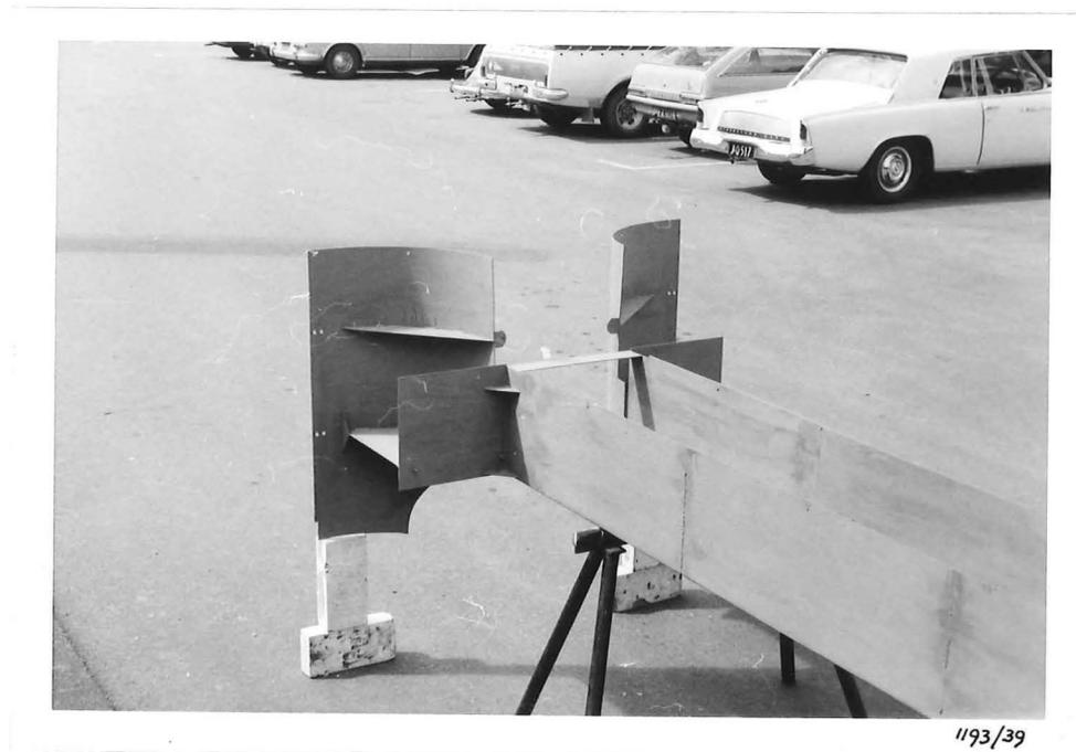
**FIGURE 5.24:** THE HIGH SPEED, FLOWING WATER CHANNEL FOR THE CONCRETE FLUME BEFORE INSTALLATION.
