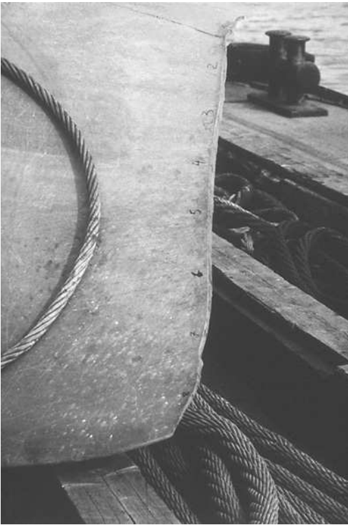
Figure 19.4 Propeller blade failure
