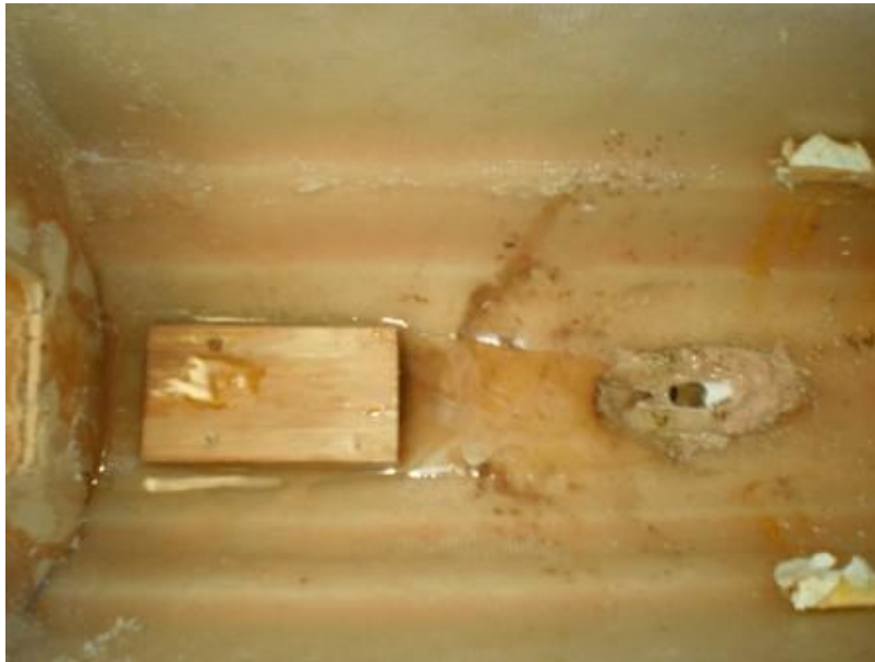
Figure 5.5.2: Original base plate in hull
