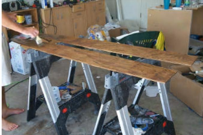
*Figure 4.2.23: Staining the decks for each hull*
