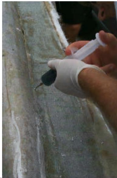
*Figure 4.2.8: Injecting resin into the air pockets between fiberglass layers.*
