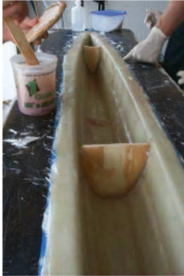
*Figure 4.2.15: Adding bulkheads to prototype using resin with a putty consistency.*
